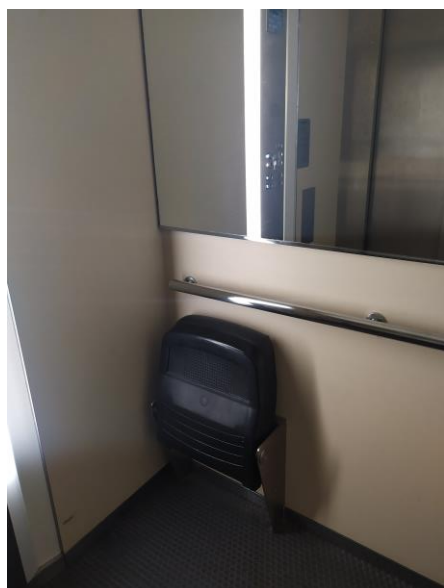
Figure 60: Lift with folding seat
