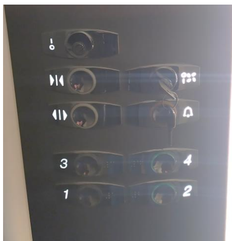
Figure 58: Control buttons in Braille
