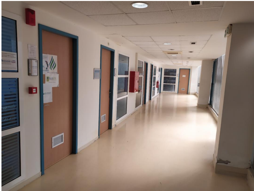
Figure 34 : Use of colour contrast at building' s internal doors
