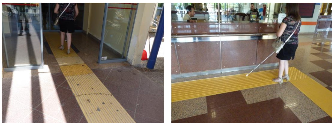
Figure 35 : Tactile surface indicators at a hospital' s entrance
