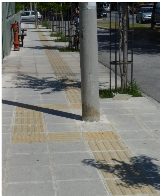
Figure 17 : Improper use of tactile surface indicators
