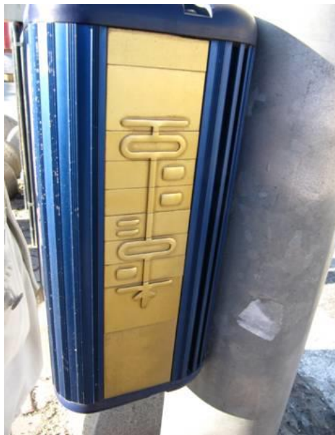
Figure 23 : Implementation of tactile indicator at pedestrian crossing
