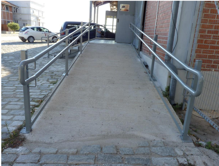
Figure 48: Ramp with proper handrail installation
