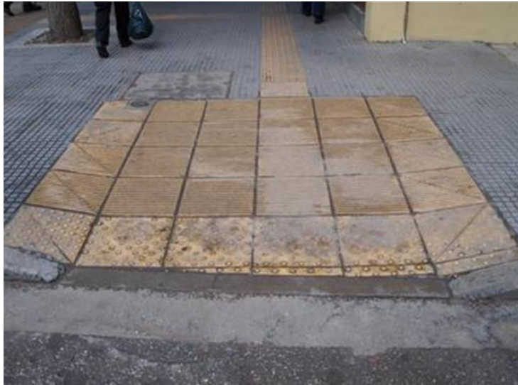
Figure 20 : Indicative ramp design
