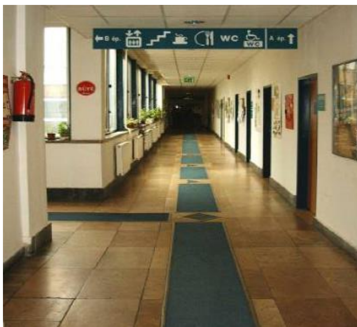
Figure 82: Internal tactile floor indicators and use of pictograms
