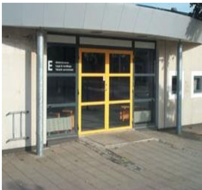
Figure 32: Application of colour contrast at building entrance
