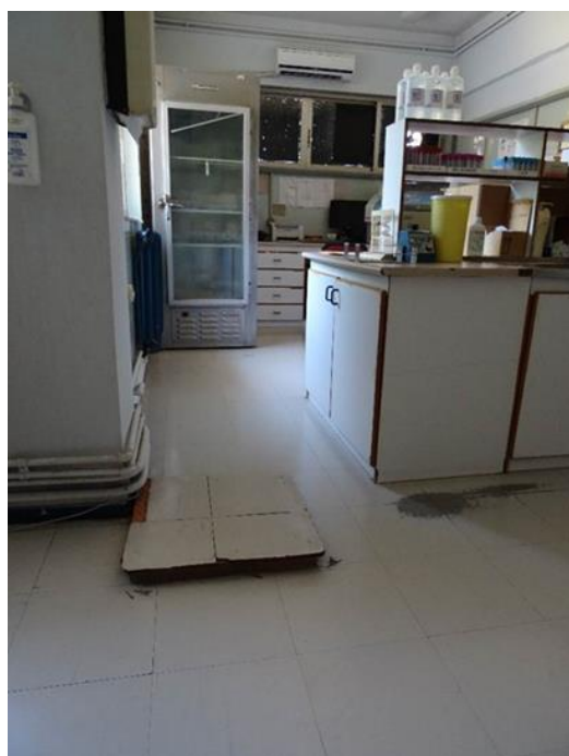
Figure 44: Protrusion at the room's floor
