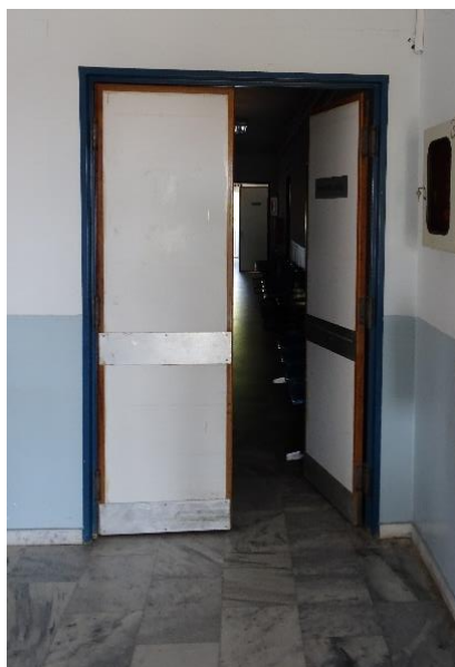
Figure 34: Internal door leading to corridors. Opening to both directions, 1,3m. clear width
