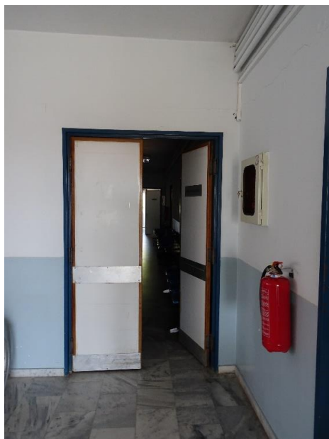
Figure 30: Internal door leading to corridors. Opening to both directions, 1,3m. clear width
