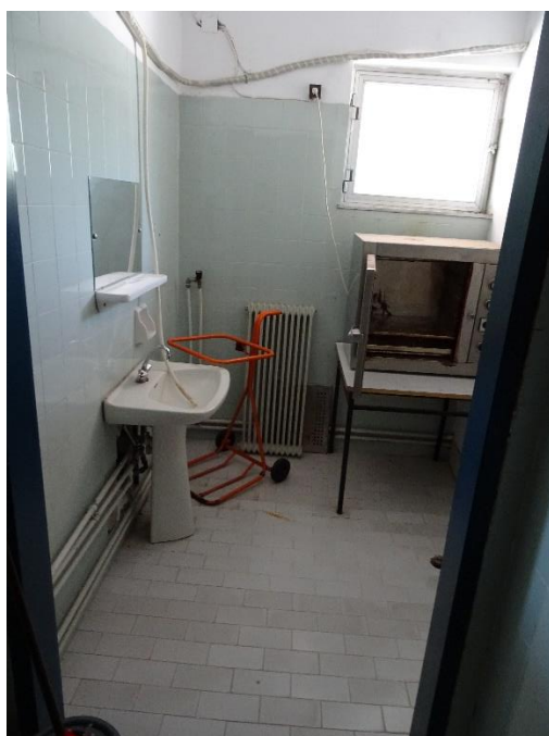
Figure 30: Rooms adjacent to the accessible toilet that can be used to increase its dimensions in case of a renovation
