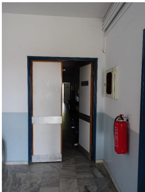
Figure 15: Internal door leading to corridors. Opening to both directions, 1,3m. clear width
