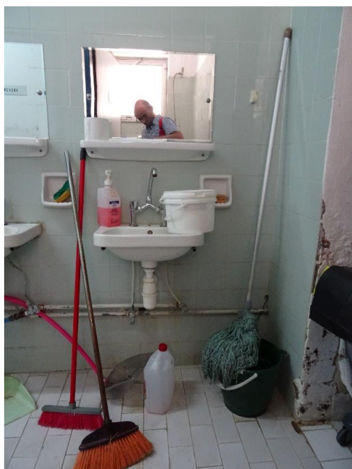
Figure 29: The washbasin opposite the accessible toilet. The free height beneath the washbasin is restricted
