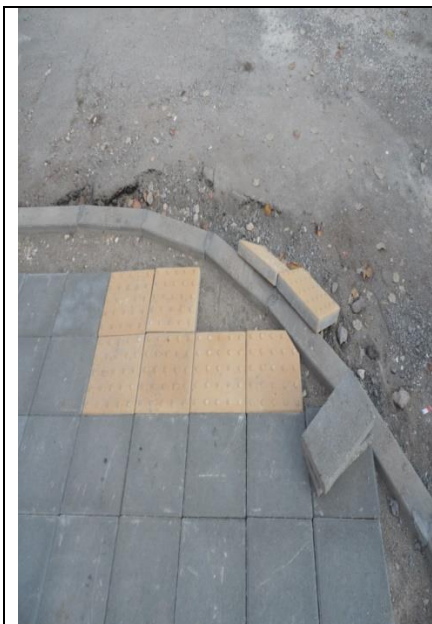
Fig. 57 Tactile indicators on renewed sidewalk
