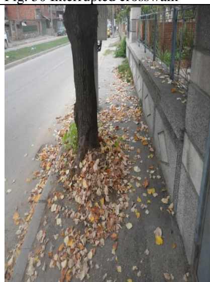
Fig. 52 Reduced sidewalk width by vegetation
