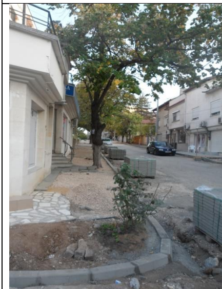
Fig. 55 Renewal of existing sidewalk
