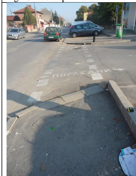
Fig. 31 Bevel, crosswalk, and parking space for disabled people
