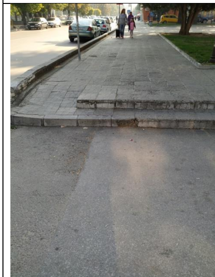
Fig. 15 Bevel and a step next to it
