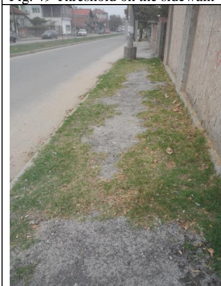
Fig. 51 Missing sidewalk flooring
