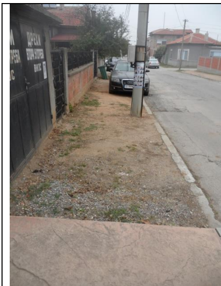
Fig. 61 Missing sidewalk flooring and parked vehicle
