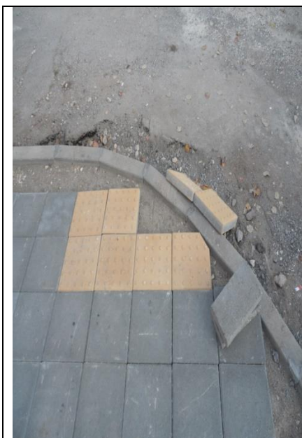
Fig. 57 Tactile indicators on renewed sidewalk
