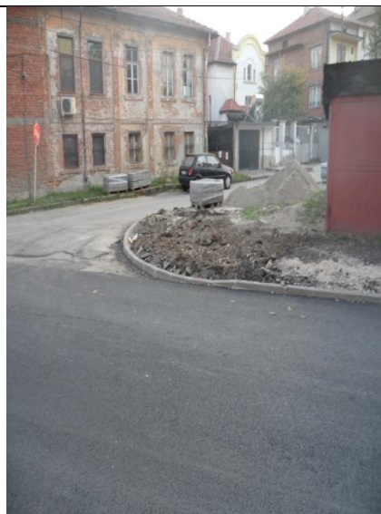
Fig. 56 Renewal of existing sidewalk
