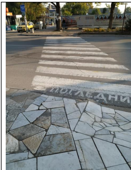
Fig. 5 Uneven flooring – marble tiles
