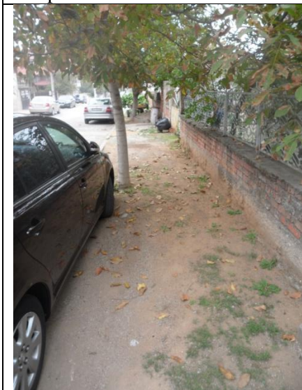
Fig. 63 Missing sidewalk flooring
