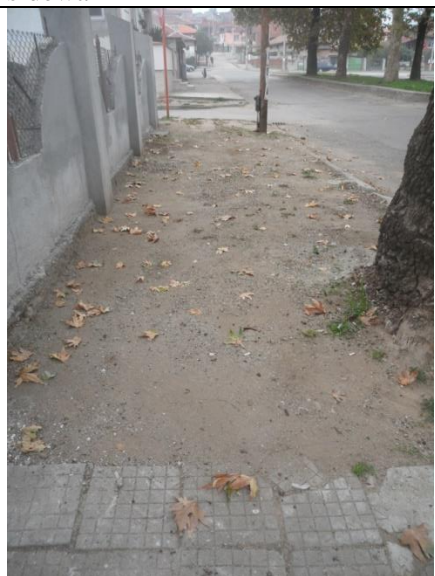
Fig. 48 Broken sidewalk flooring
